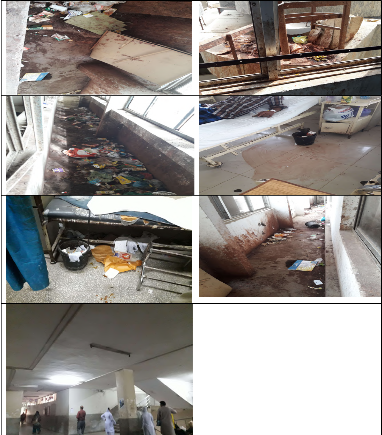
Sanitation and Lighting System
